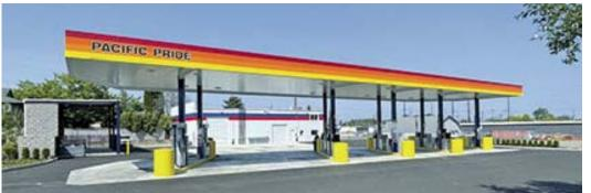
Marc Nelson Oil Products has rebuilt its Pacific Pride cardlock and bulk fuel facility in Gresham, OR. Located at 150 NE Hogan Drive, the project expanded the cardlock, upgrading equipment, and converting the bulk fuel facility from top-loading to bottomloading. There are four diesel fueling positions with three having master and satellite dispensers
